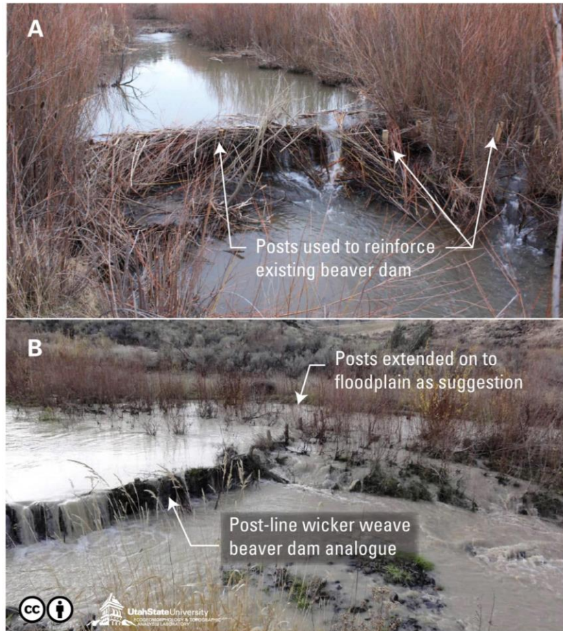
Figure 1. Reinforced natural beaver dam (A) and human-constructed BDA (B). Reprinted from Shahverdian et al. 2019.
