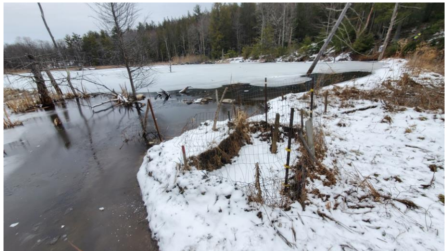
Figure 6. View of the impoundment, looking north. At the foreground, fencing protects the flow leveling pipes installed by the property owner. February, 2023.
