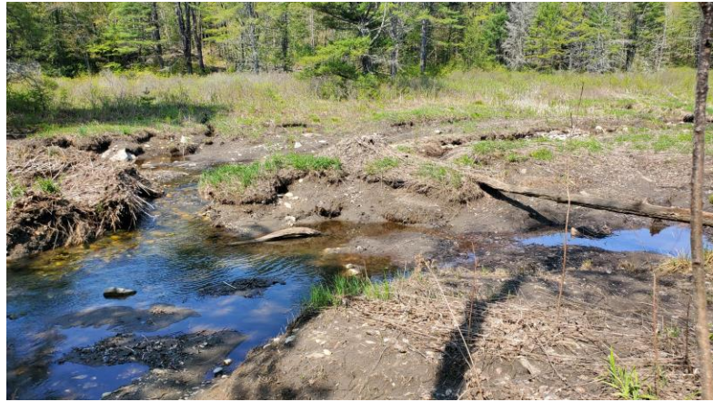
Figure 12. View of the former area of impoundment along Kinne Brook as observed in May 2023. Areas of bare soil indicate the extent of the impoundment prior to dam breach.
