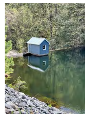
Figure 4. Dam at Horn Pond.
