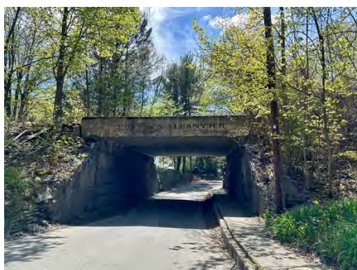
Figure 6. Boston & Albany R.R. Bridge in Chester Village.
