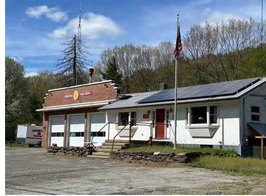
Figure 5. Chester Fire Station.
