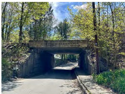
Figure 6. Boston & Albany R.R. Bridge in Chester Village.
