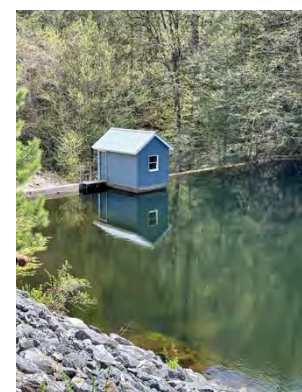
Figure 4. Dam at Horn Pond.
